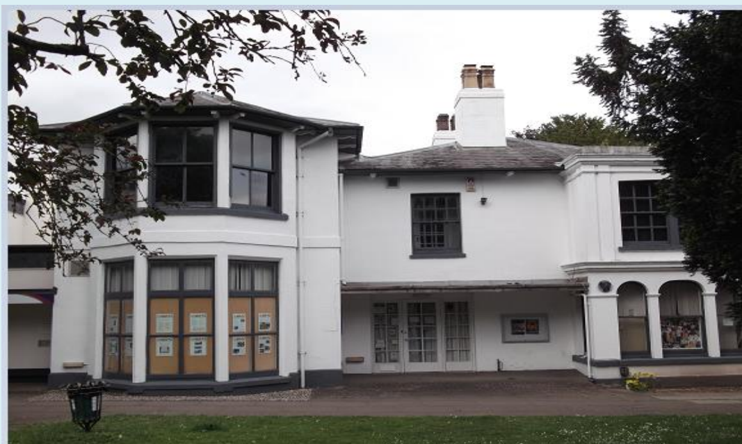
Charnwood House: Front (south-west) elevation. Photographed 11 th June 2021
